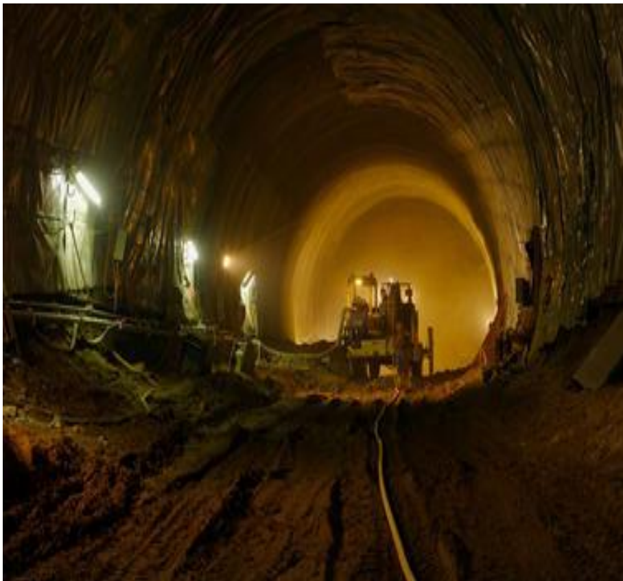
Figure 4: Construction works metro tunnel U55
