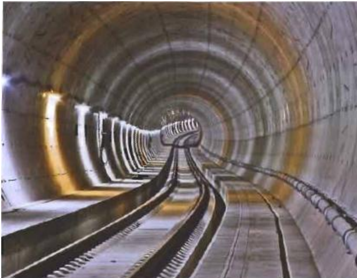
Figure 2: View into North-South railway tunnel tube constructed with tunnelling shield
