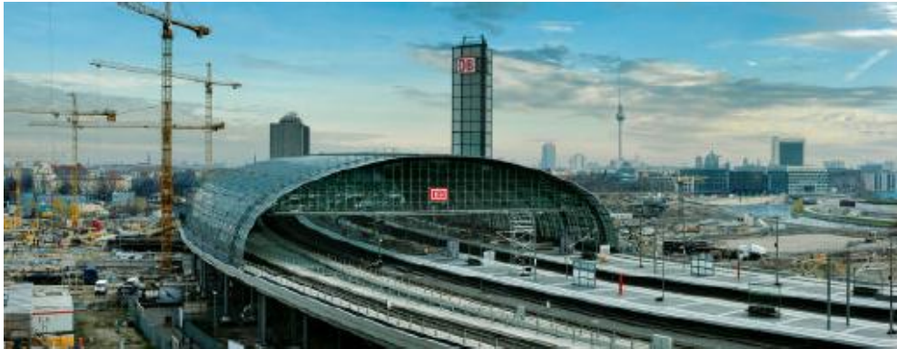
Figure 9: Berlin Central Station under construction
