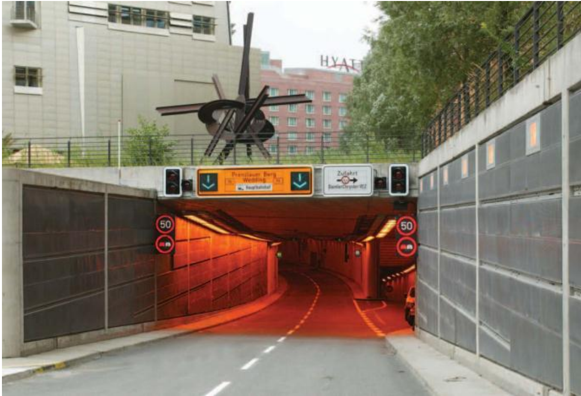
Figure 1: Entry of the car tunnel in the South near Landwehr Canal
